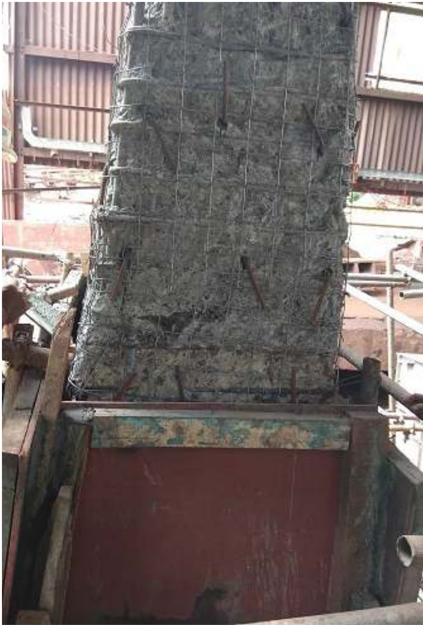
Essar Port Complex Column Base
